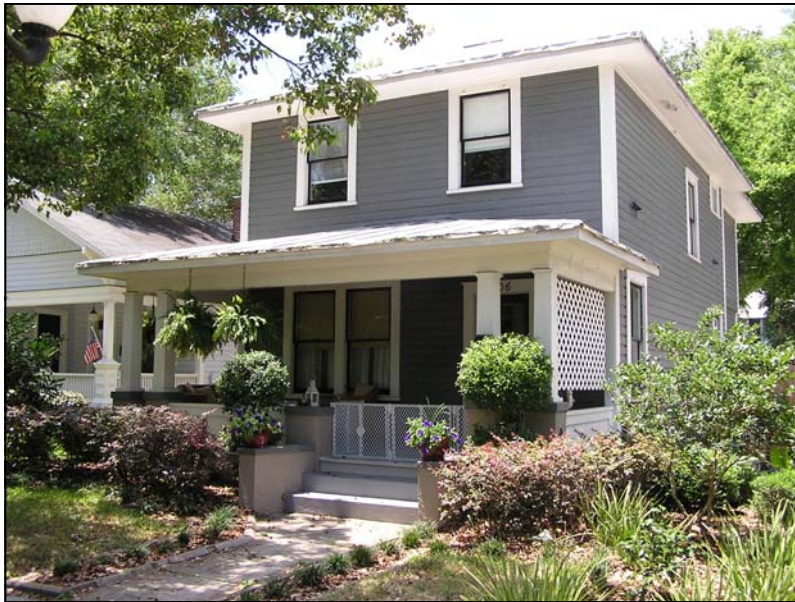
706 Palmetto Avenue, Circa 1917 Architectural Style: Frame Vernacular, National (Pyramidal) Residential Historic Preservation Award
